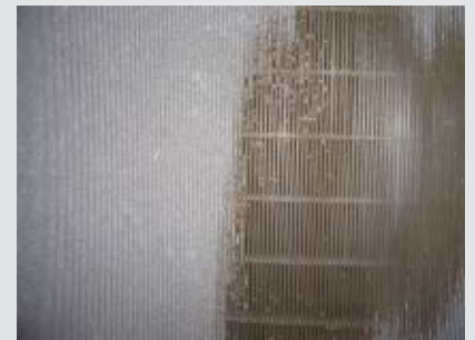
Photo - CCR Regenerator Clean
