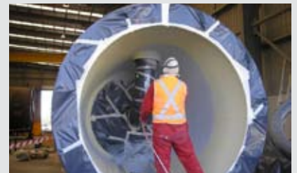
Photo - Tom McCormack fireproofing a vessel at Pipetech Engineering, Adelaide SA.
