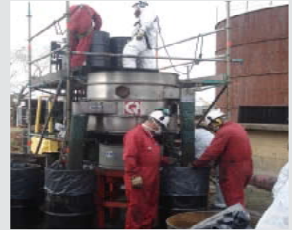
Photo - Screening of the spent catalyst and inert balls prior to reloading.
