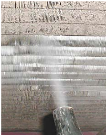
Photo - Cleaning effect of Decamex on fin fan bund
