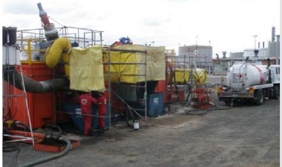
Photo - Peter 'Google' Welch utilizing a custom made hopper for decanting catalyst
