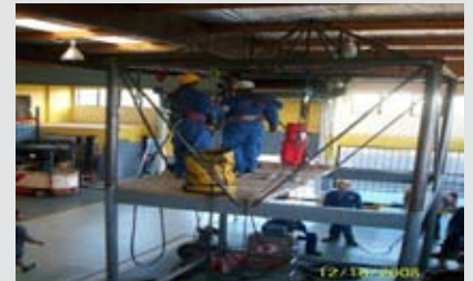
View of Vertical Horzionz working at height Platform
