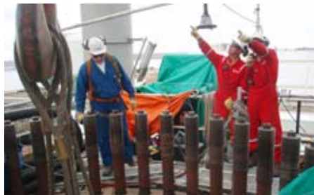
Photo (Top) - Ammonia converter in Profertil. Preparation for the removal of the top basket
