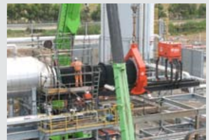
Photo - Crew loading Catalyst bags into Dense Loader surge hopper
