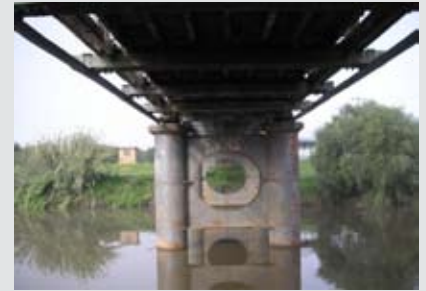
Photo - Before painting on piers
