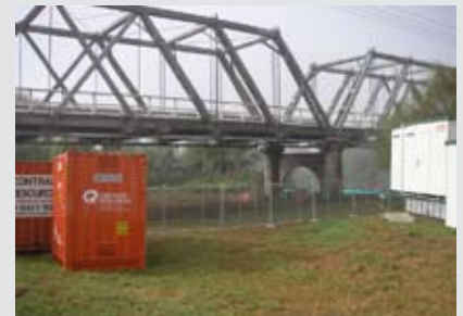
Photo - Showing area near bridge that flooded with recent rains
