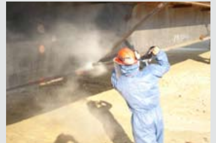
Photo - Nathan Gribben undertaking test blasting to ascertain remaining sodium levels
