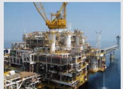
Photo - The Drilling and Production Platform (DDP) where Chemical Cleaning, Hydro Jetting and Vacuum drying works were carried out during the Bayu Undan Shutdown.
