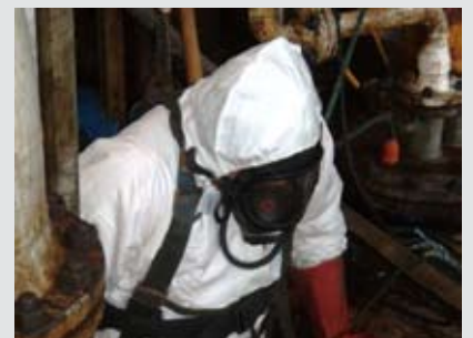
Photo - Contract Resources Crew during the sludge removal process
