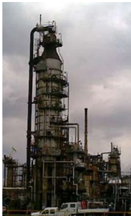
Photo - The beast - 2C1 conquered by CR's mechanical and cleaning crews.
