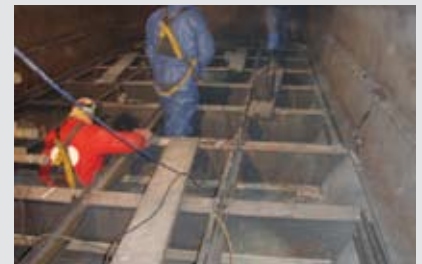
Photo - Carrying out modifications during the Port Kembla project
