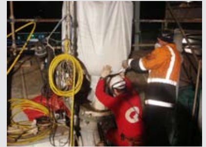
Photo - loading last of material on the Port Kembla project
