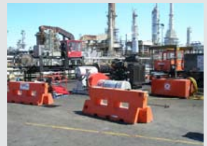
Photo - The HPW waster blasting pad
