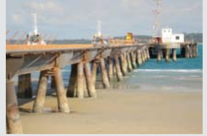
Photo - Cargo Wharf - approx 300m long
