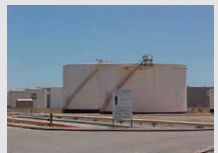
Photo - the tank located at Mobil Altona where CR personnel commenced work late November
